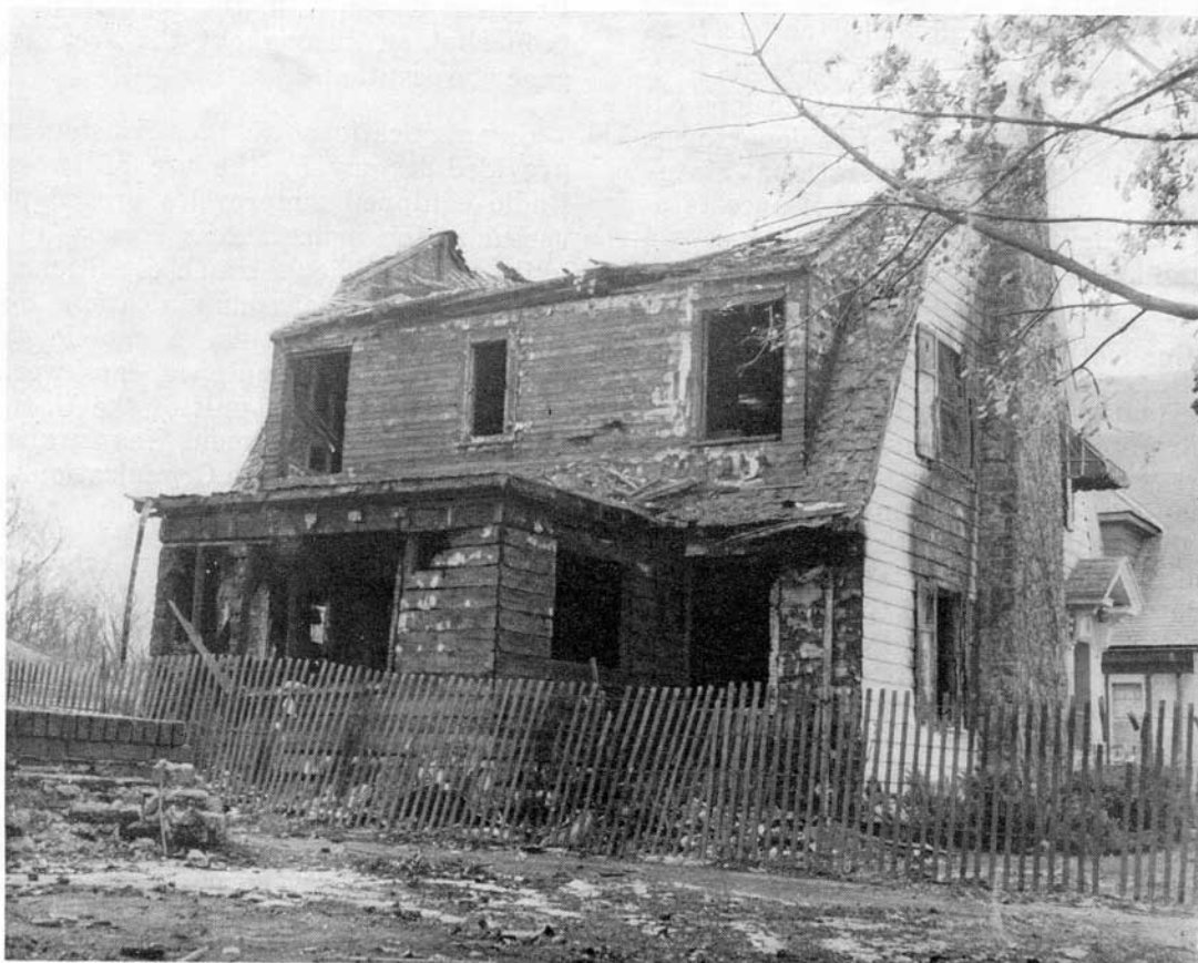
FIG. 20. Another example of fire exposure damage on Mayflower Drive.
