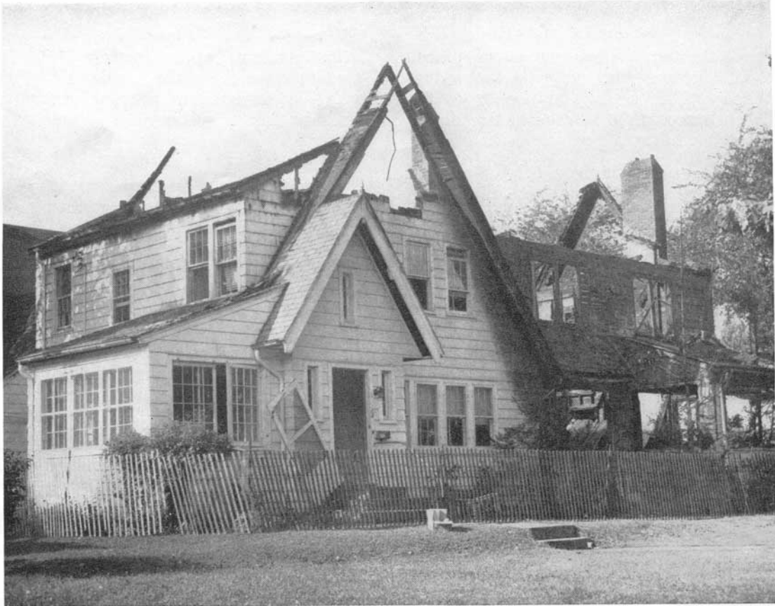
FIG. 17. Damage to this two-family dwelling at the corner of Sylvan Road and Fair Oaks Avenue was limited by a dividing wall extending only to the attic.
