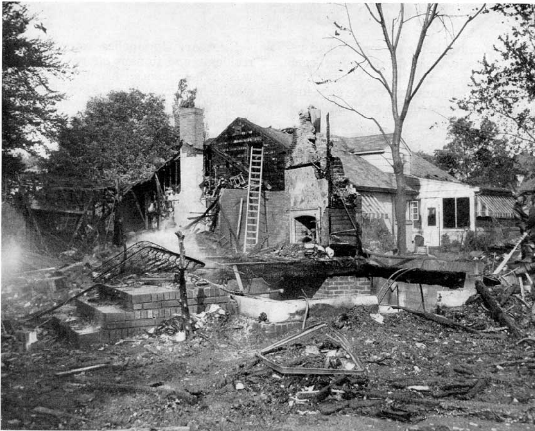
FIG. 19. Effects of explosion and fire at Oakdale and Mayflower Drives.
