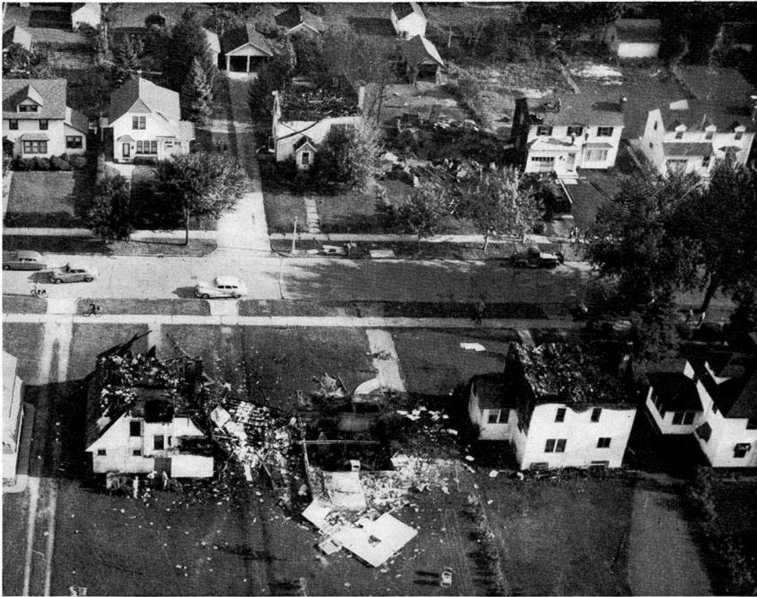
FIG. 11. Antlers Drive—Houses destroyed by explosions and damaged by exposure fires.
